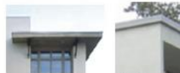
Cantilevered roof planes
