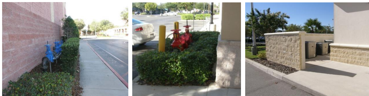
Figure 26: Screening of Equipment/Utilities
