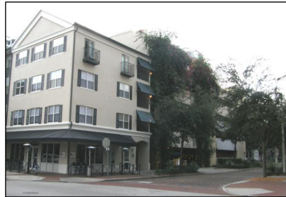
Parking structure behind liner building
