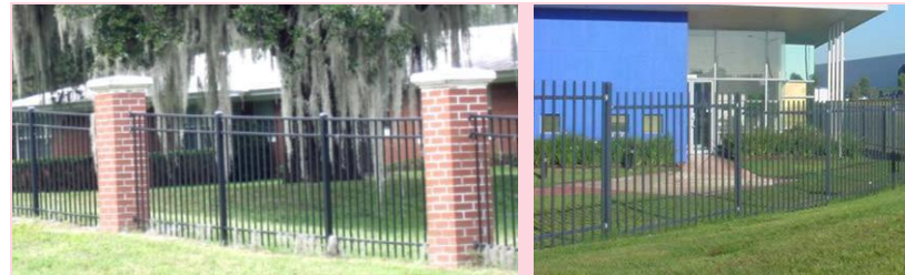
Metal picket fencing alongside/rear yards
