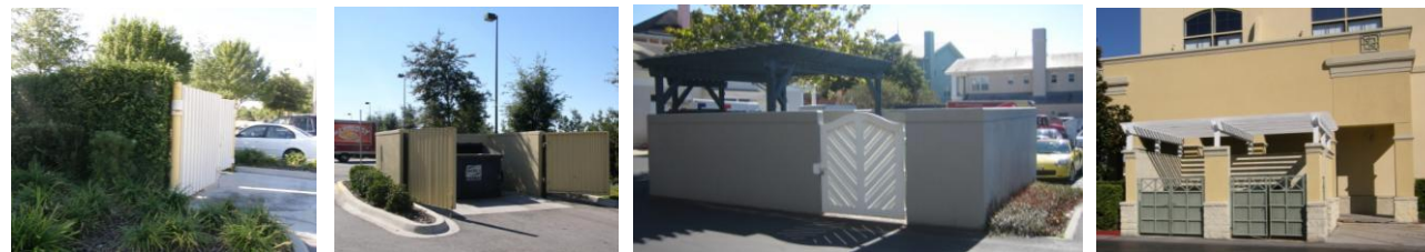
Figure 28: Screening of Trash Containers
