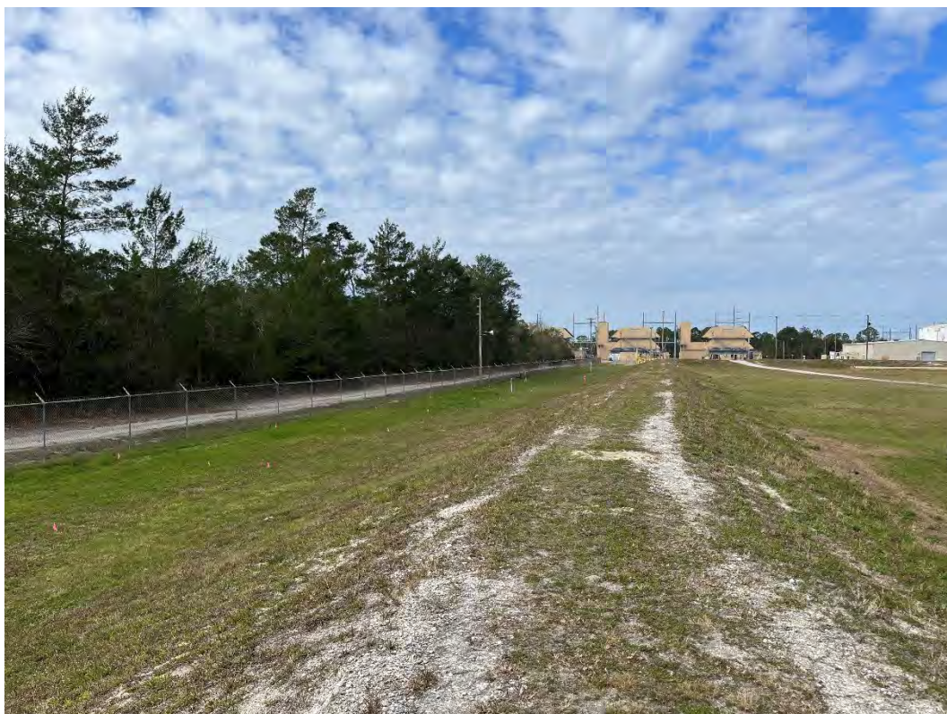
Photo 2. View of the Site looking West Along Southern Berm
