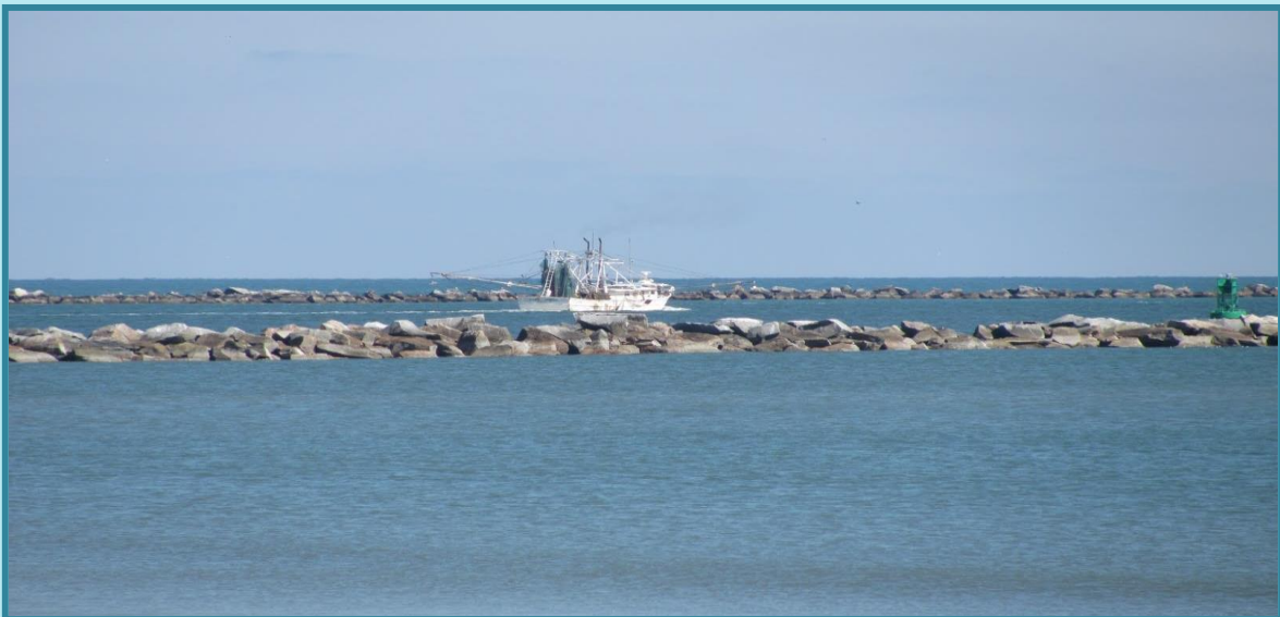
JETTIES Mayport Naval Station
