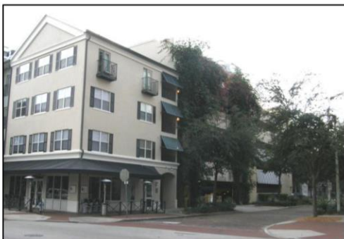
Parking structure behind liner building
