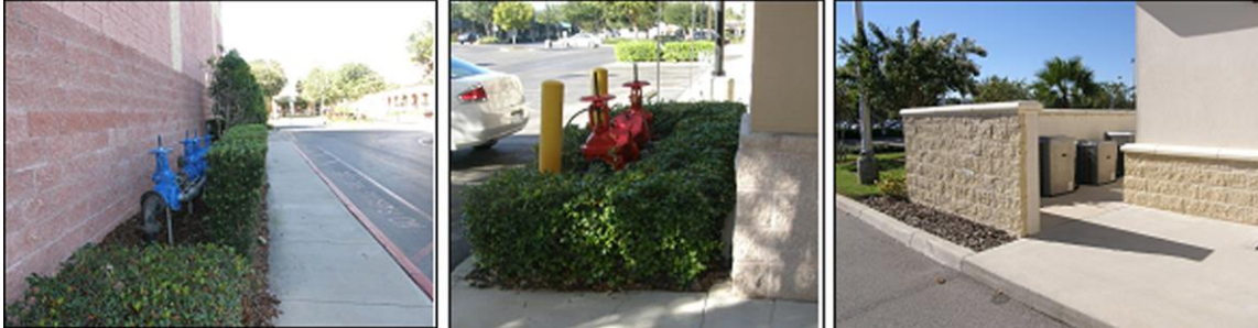
Figure 5 - 74: Screening of Equipment/Utilities
