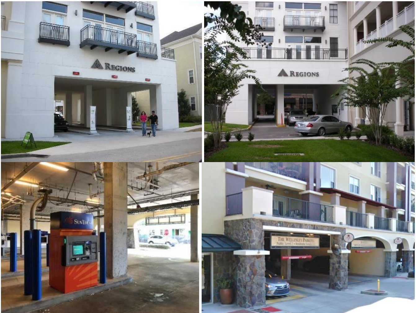
Figure 5 - 36: Interior Drive-Through Facilities
